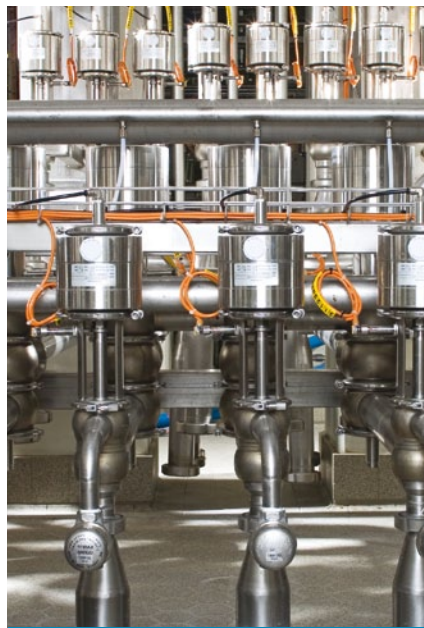
Fruit tank top valve matrix
