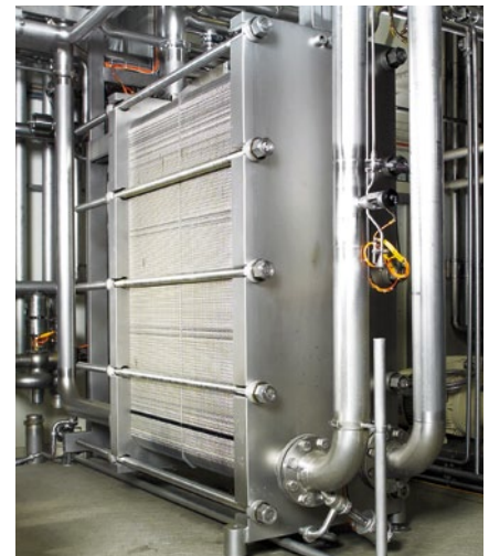
Plate heat exchanger with a capacity of 50,000 l/h
