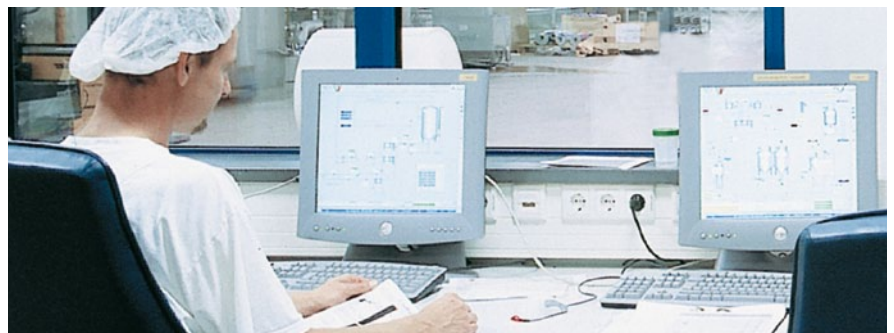
Central control room
