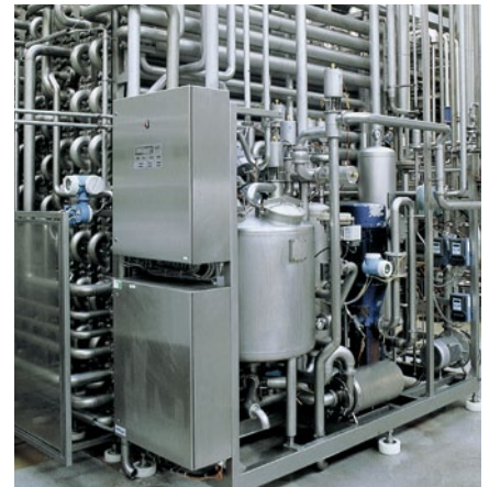
STH Plant (RWT) for fruit juice, capacity 20 m 3 /h
